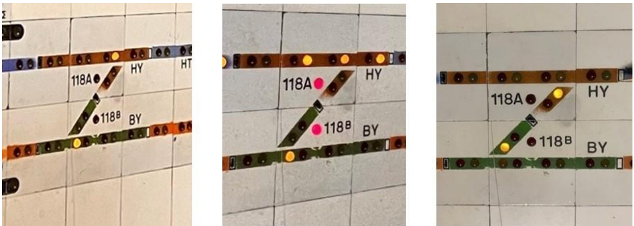
Figure 47. Detail of the switches 118 on the Larissa Control Panel (main-moving-bypass).
