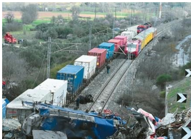
Figure 84. Positions 8)-15) The remaining platforms carrying 8 containers, undamaged and still sealed (or remained empty, of the 2 last ones), not derailed, stopped along the line and were driven away normally.
